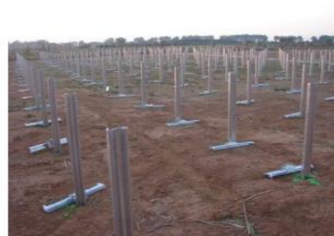
Aspect des supports
